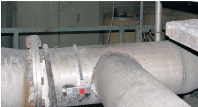
Strap-on ultrasonic sensor is not affected by the abrasive and caustic fly ash slurry
