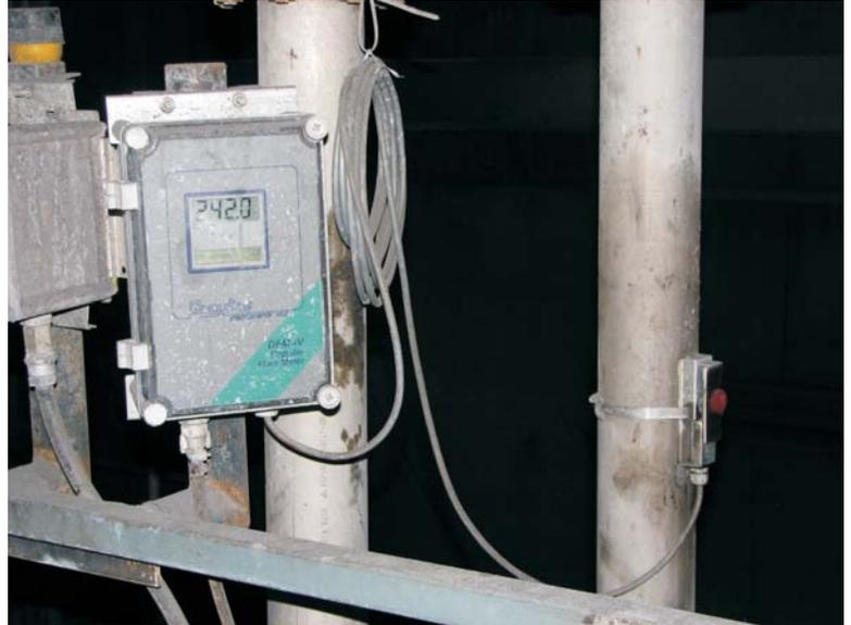
Greyline DFM-IV Doppler Flow Meters installed to measure "fly ash slurry" at Xcel Energy's Sherburne County Generating Plant in Becker, Minnesota
